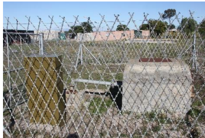
Riverlands BH No.2, fenced and locked
