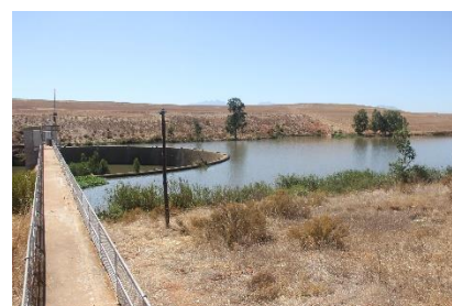
Misverstand Weir: Supply to Withoogte WTW
