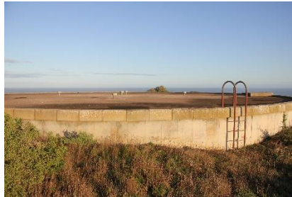
Yzerfontein Reservoir No.2, 2.553 MI
